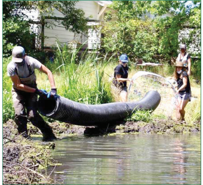
Flow control device for beaver dam
